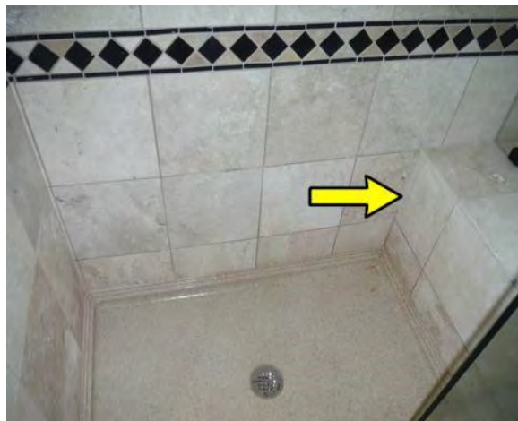
Reseal around base and corners as required in the master shower.
