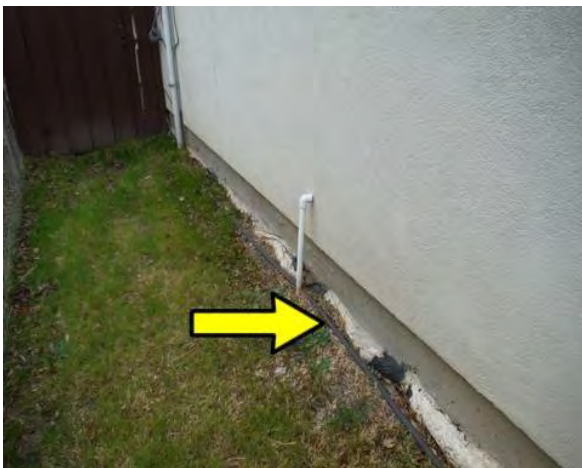
Foundation beam exposed on west side.
