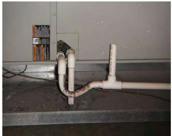
Example of correct installation of p-trap and vent on main condensate drain line.
